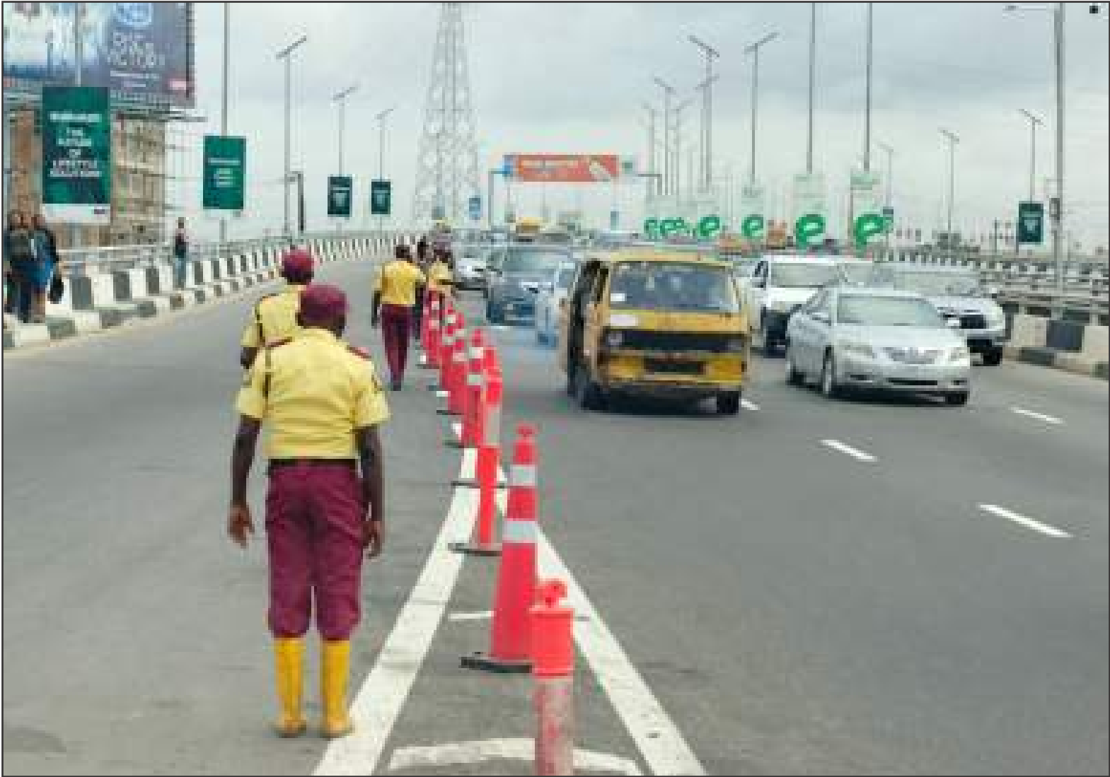
2nd Phase Ogudu-ifako bridge
