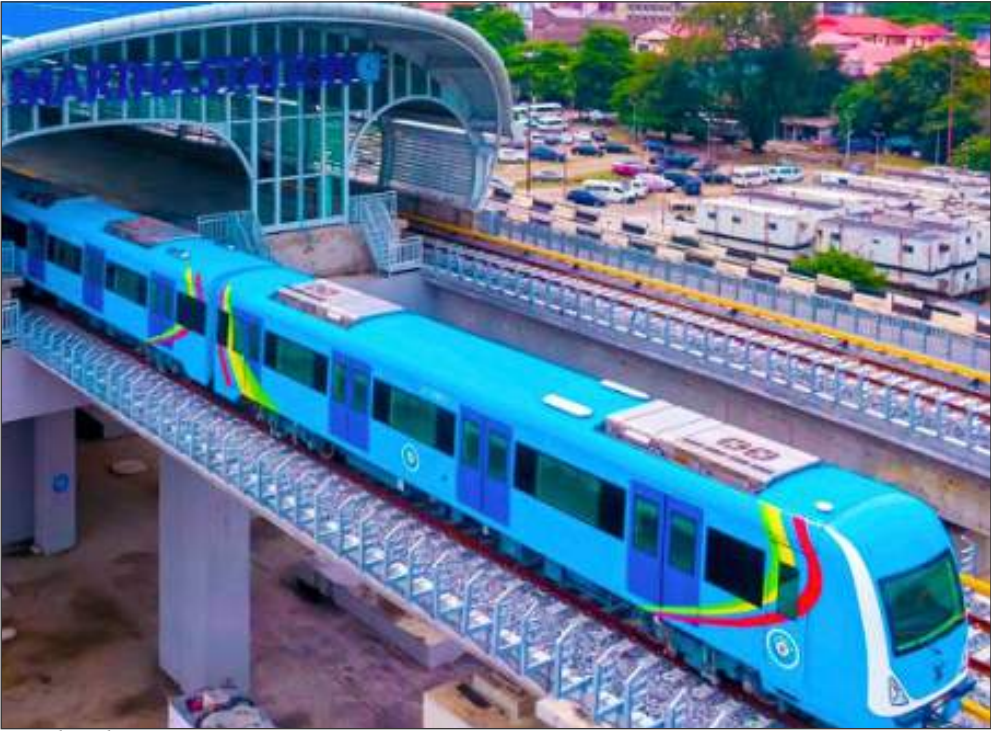
Lagos Blue Rail Line
