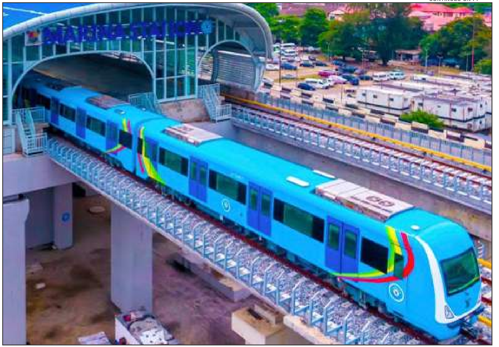
Lagos Blue Rail Line
