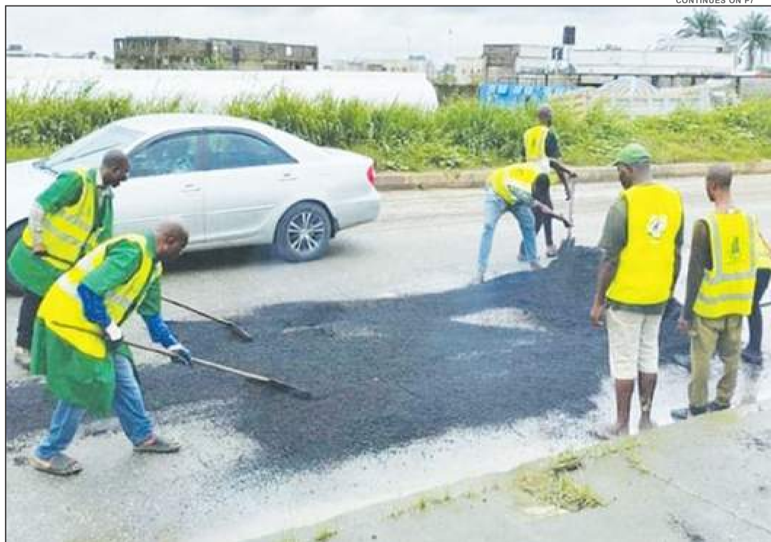
FERMA workers working on a road project
