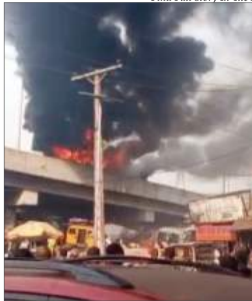
the fire on the BRT bus
