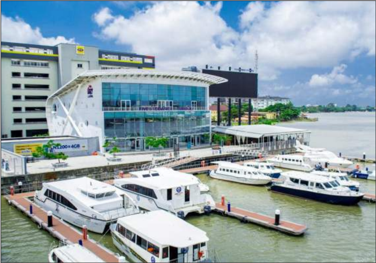
Lagos State Waterways Authority (LASWA) Headquarters at Falomo
