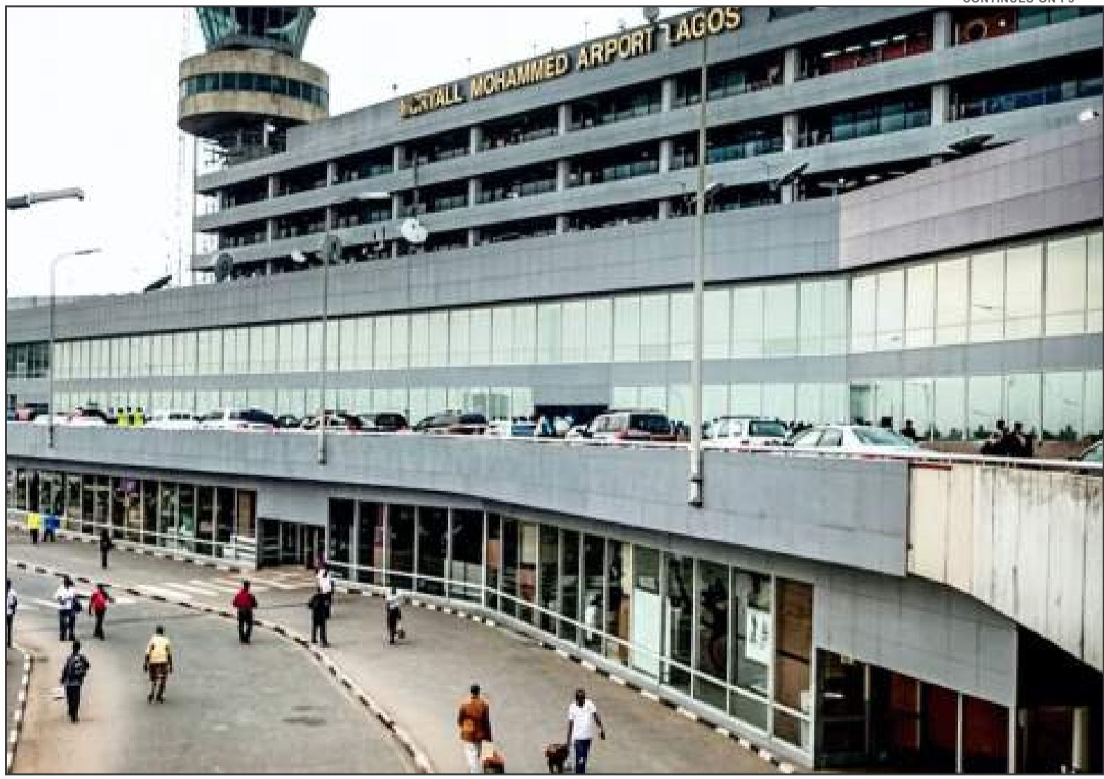
The Muritala Mohammed airport, Lagos
