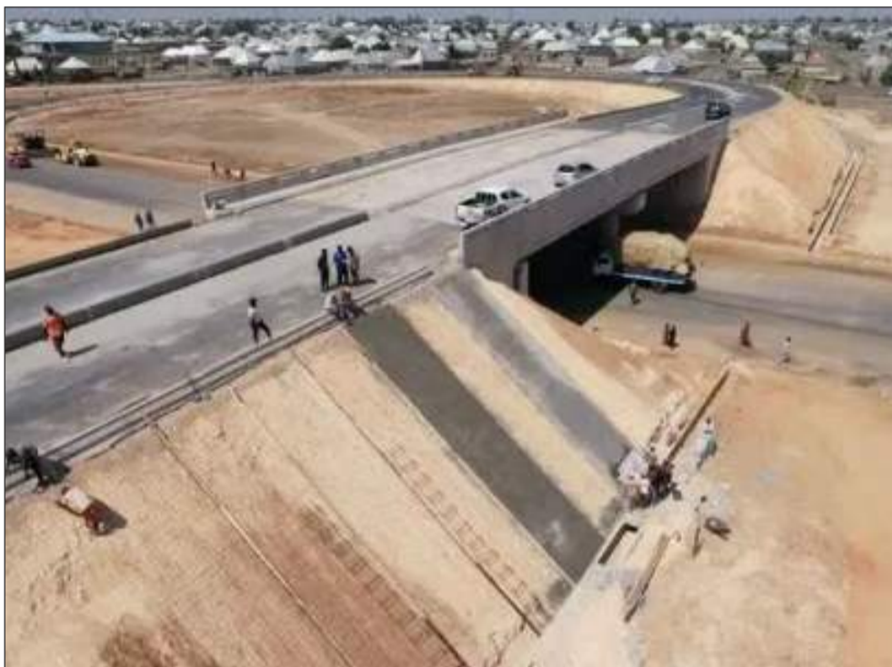
The Bauchi-Gombe road reconstruction
