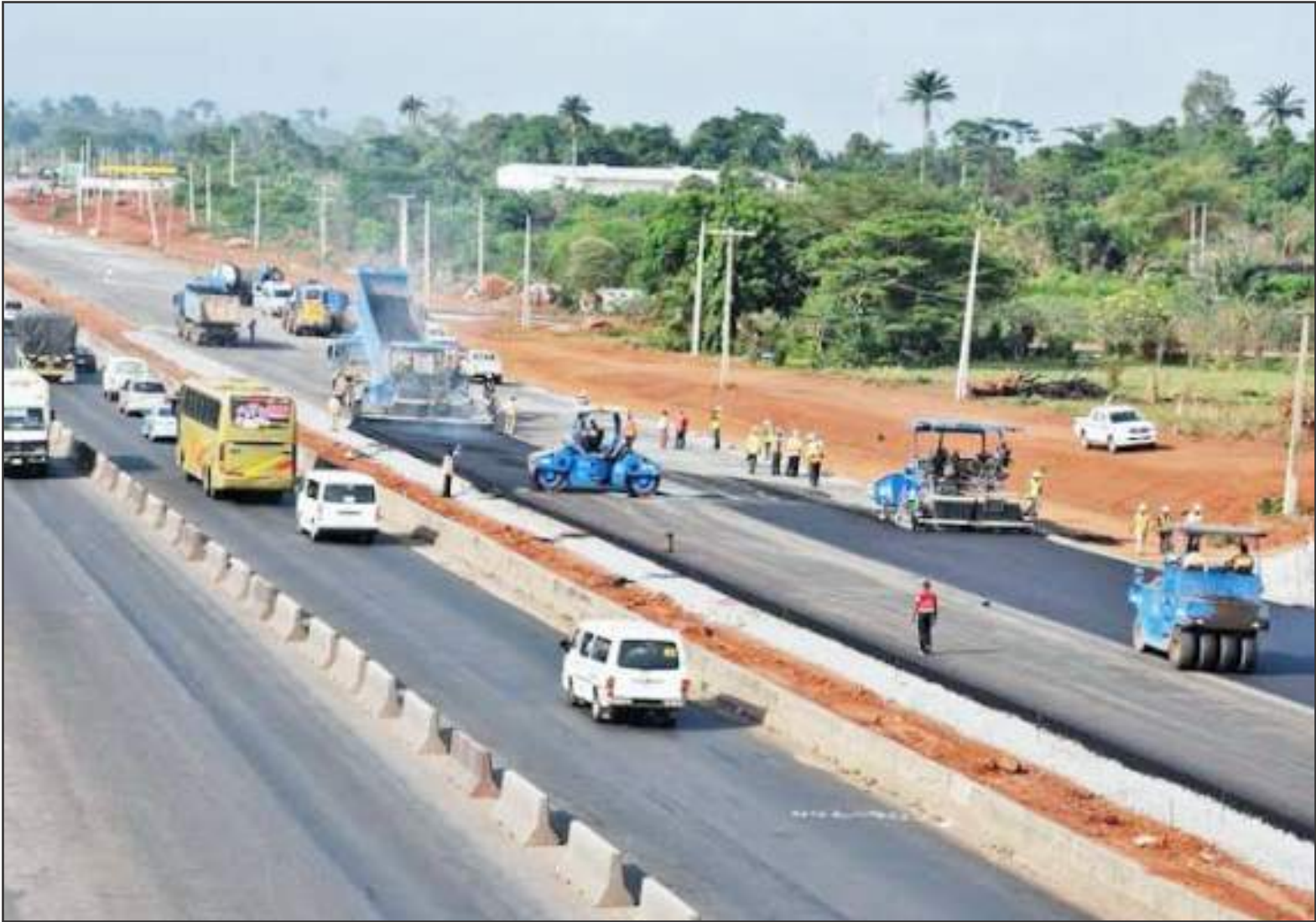
Traffic diversion on the Lagos-Ibadan Expresway
