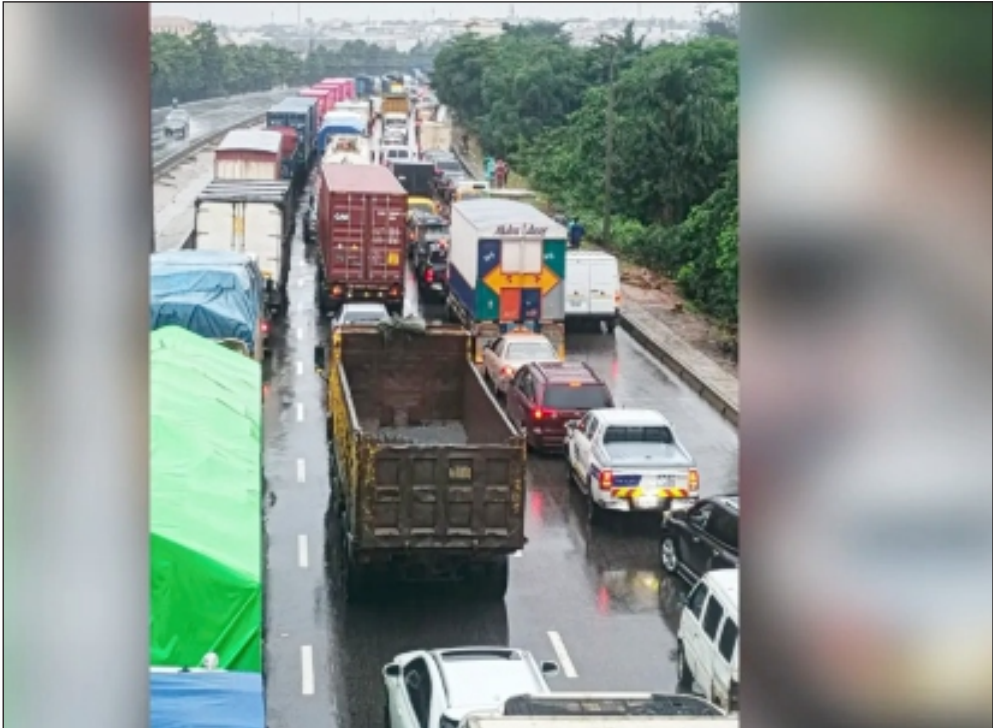
Fast track repairs on the Kara Bridge
