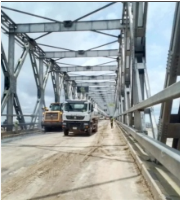
The First Niger Bridge
