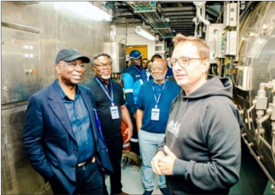
Dr. Mobereola on a working visit and inspection tour of Marine Platforms Limited
