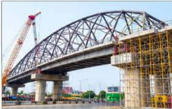
The ongoing Opebi-Ojota link bridge project in Lagos.
