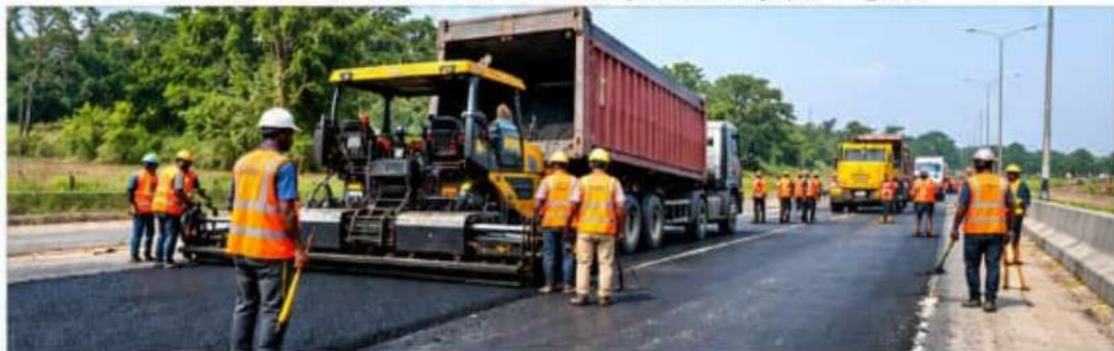
Construction work in progress on a federal highway project in Nigeria, on Wednesday.
