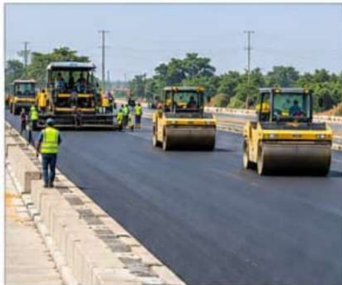
Road construction works on a federal highway section in Nigeria.
