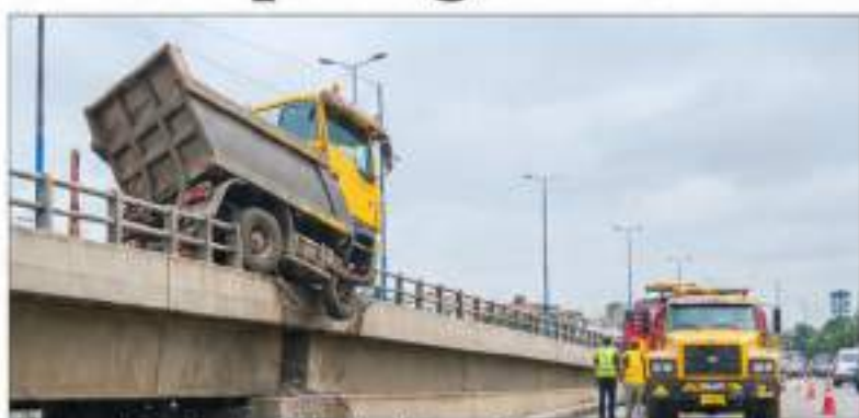
A tipper truck hangs from Kara Bridge along the Lagos-Ibadan Expressway.
