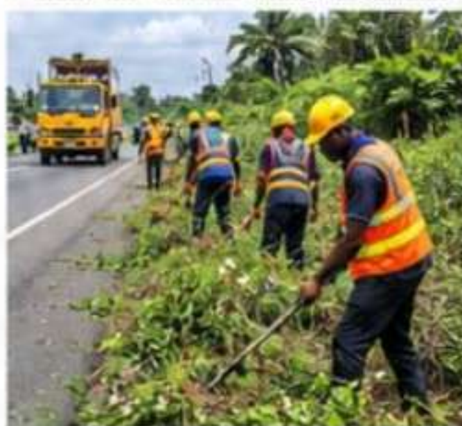
FERMA maintenance work targets safer visibility and drainage along the Calabar-Atimbo-Ikang road.
