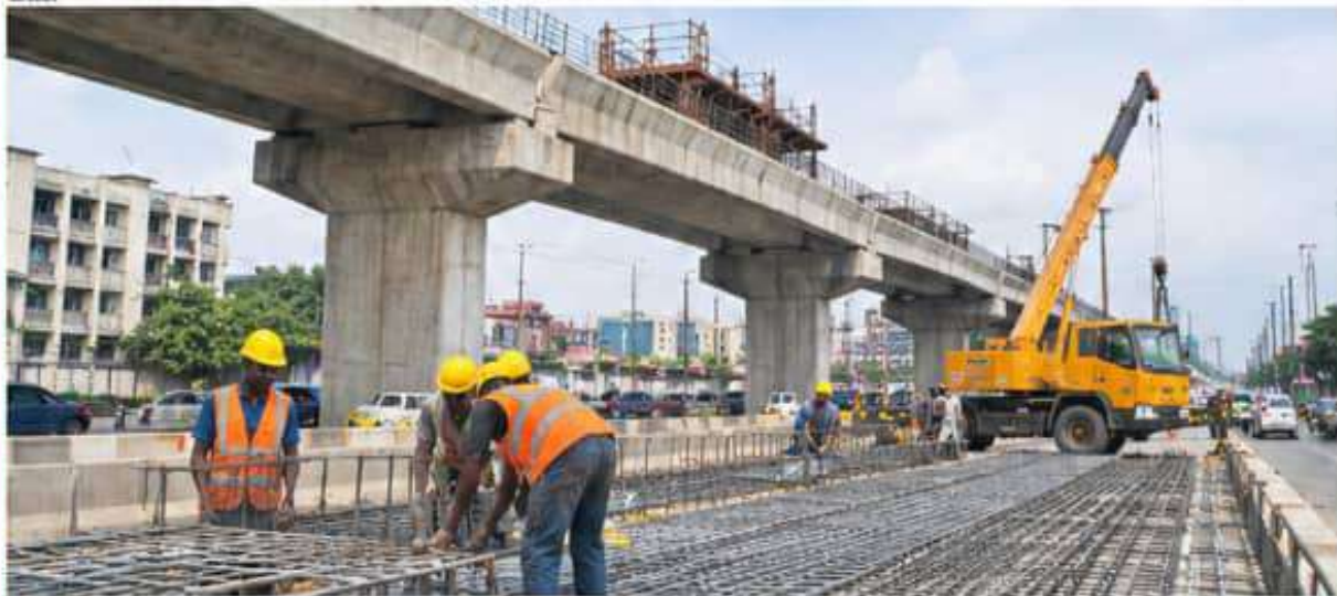
Ongoing construction work on the Opebi-Ojota link bridge, Lagos, on Monday.
